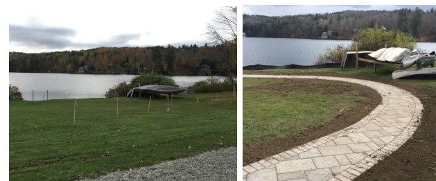
Before and During Construction Permeable Pavers to Manage Stormwater Silver Lake State Park, Barnard
