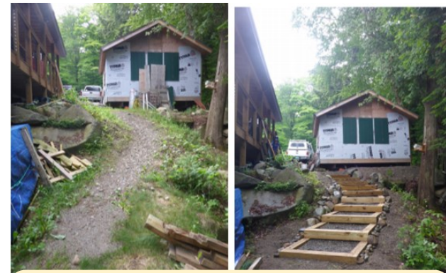
Before and After Infiltration Stairs to Manage Stormwater Maidstone Lake in Maidstone
