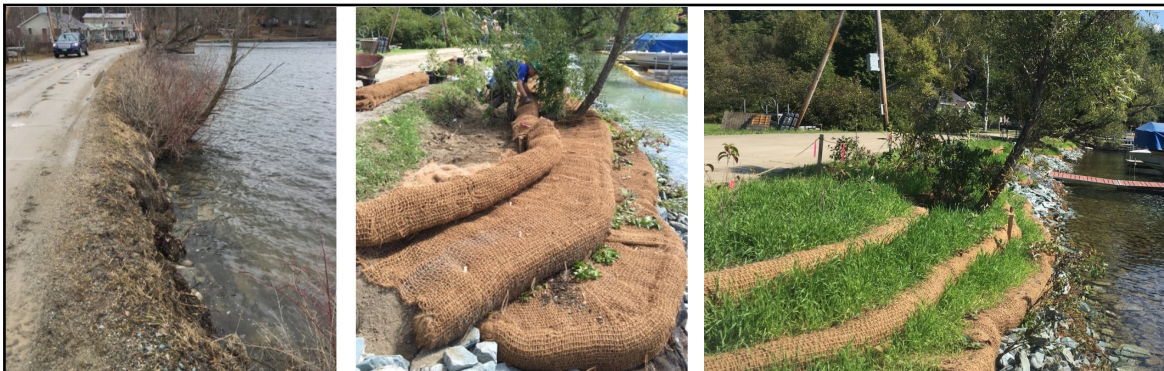
In 2017, the Town of Castleton stabilized 300 feet of shore along Lake Bomoseen Funded by VTrans Better Roads Program
